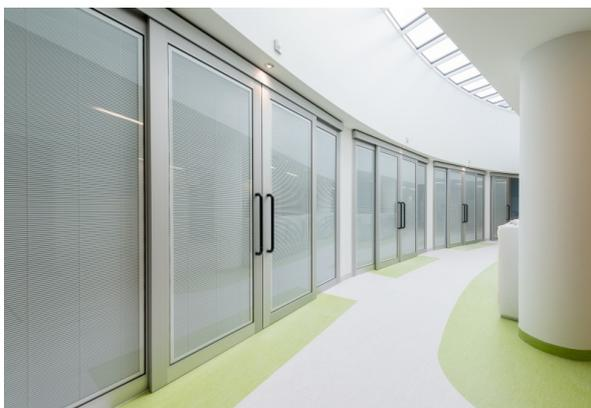
In response to these challenges Axis developed a unique top hung system with an integral soft-close dampening mechanism applying a true R&D approach. As a direct result of the door design, all patients have excellent views of the nursing team providing their care and vice versa. The glazed wall and door
