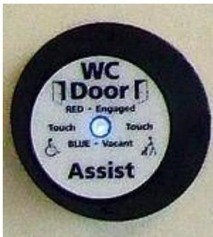
**Stage 1** - the external touch entry sensor is activated and the door opens.
